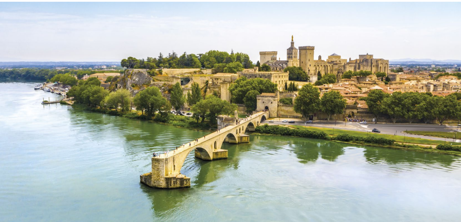
St Benezet Bridge, Avignon, France
